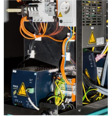
*Caption 2: The client-specific buffer module in the centre of the image serves for supplying additional power during peak loads and is recharged using the modified QT40.241.*
